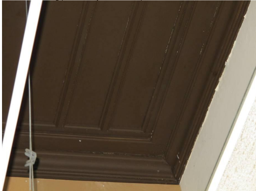
Detail plafond. Foto FH MAB 2013
